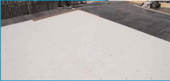
F - The screw locations are pre-marked on the boards
