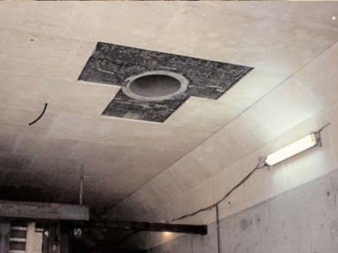
Openings for manholes can easily be made by using phenol coated plywood panels
