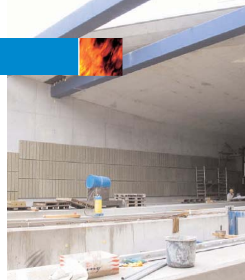
Aquaduct Abcoude, Netherlands
