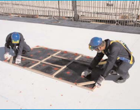
Template for screw location
