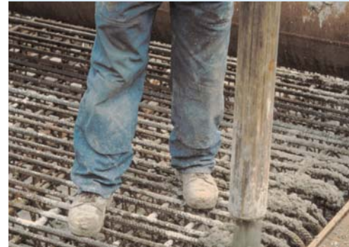
K - The pouring of the concrete
