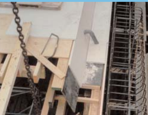
Inclusion of services and pipes in formwork
