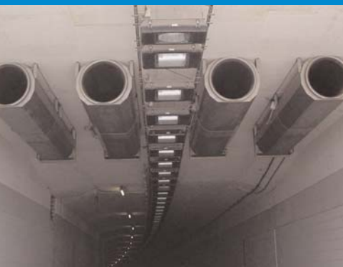
Anchors for services are installed through boards into the concrete, thus creating a continuous fire protective layer
