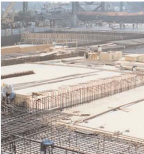
Harbour Tunnel CANA, USA
