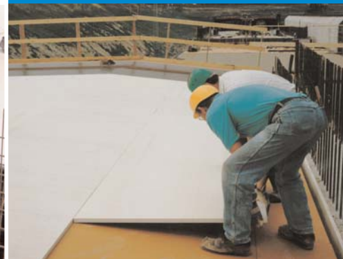
Distance between formwork and wall, easing the extraction of the formwork
