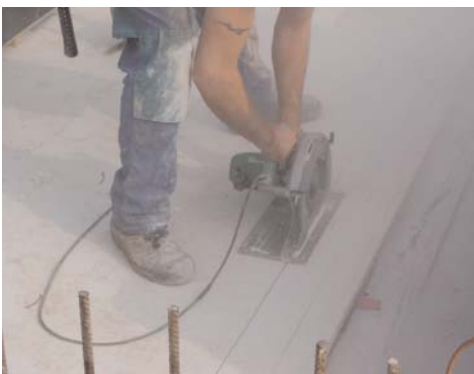
Cutting the boards on the formwork eliminates the tolerances
