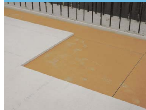
Regular load bearing plywood can be applied, instead of phenol coated plywood
