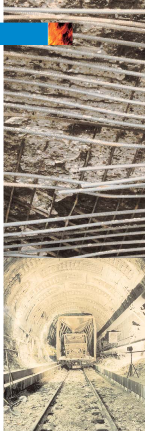
Severe concrete spalling after fire exposure in tunnel
