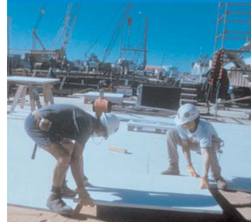
City Northern Bypass Tunnel - Perth, Australia
