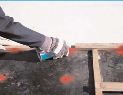
Spray can to mark screw location using template
