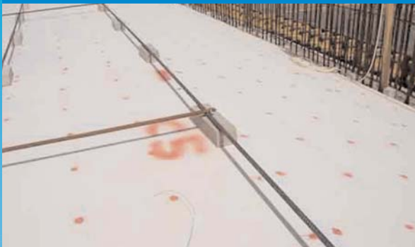
G - First layer on reinforcement installed, prior to inserting the screws
