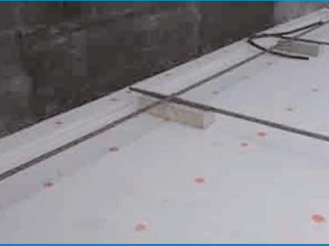
Detail of an expansion joint and cover strip allowing movement
