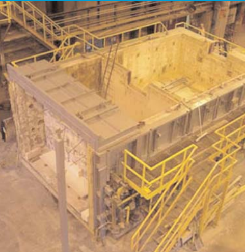
TNO Efectis Netherlands: largest RWS-fire capable furnace in Europe
