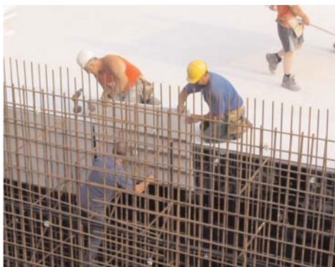
Wall panels can also be installed using the lost formwork method
