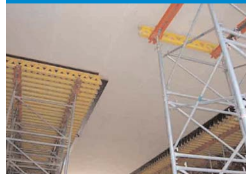
L - Extracted formwork. Flush finish of the ceiling
