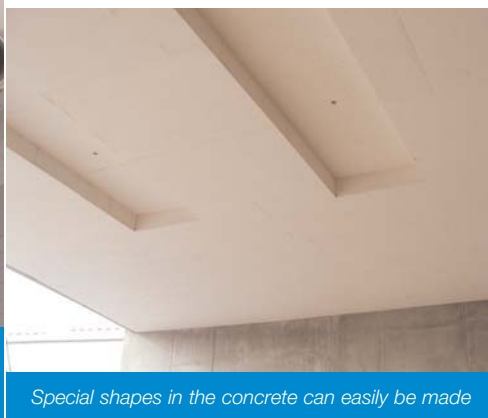
Anchors for services are installed through boards into the concrete, thus creating a continuous fire protective layer
